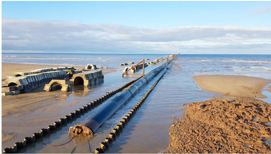
Plate 3: Example of a pipeline within a sheet piled trench prior to being submerged and backfilled. Note the concrete anchor collars.
